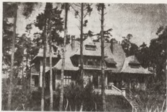
ONE OF THE NEWLY ERECTED STANDARD COTTAGES IN THE STATE FORESTS
