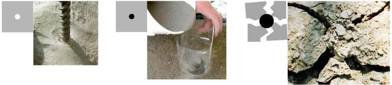
**Fig. 9.** Phases of the technological process of splitting rock solids with the use of expanding materials [22]
